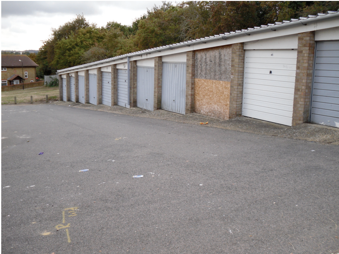
Plate 4. Detail view of the existing garage block on the proposed development site (facing south-west).
